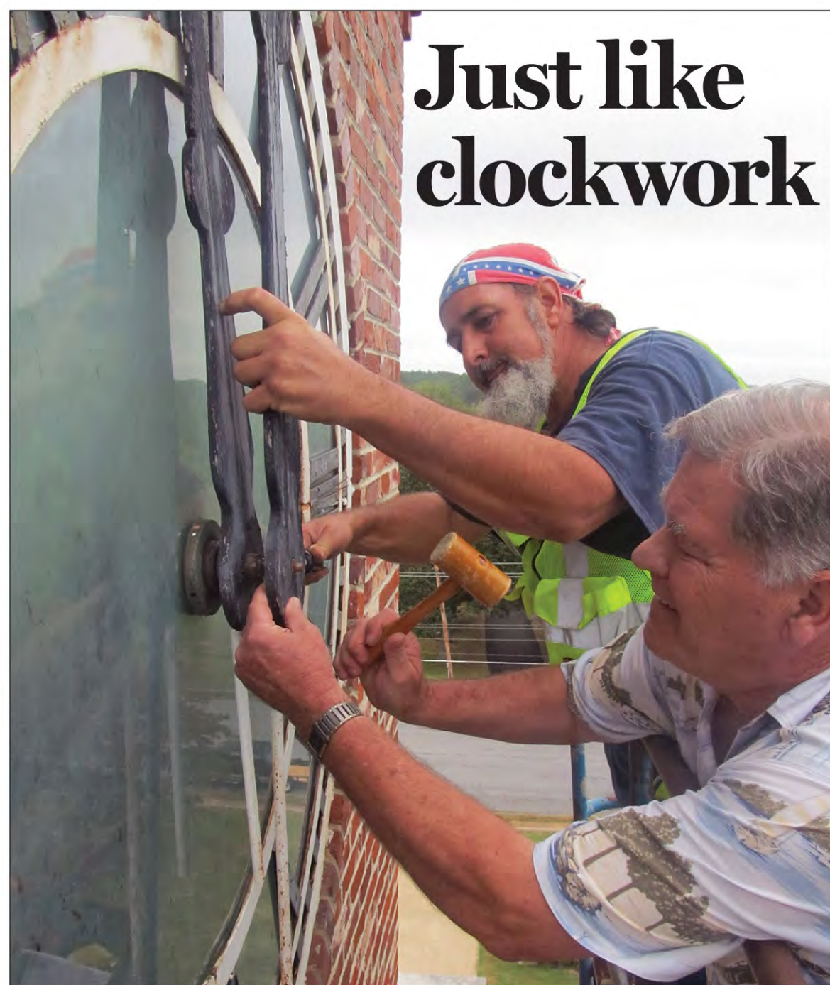
Clock repairman Jim VanOrsdel, right, receives assistance from Cliffside resident James Harris, middle, in removing the hands from one of the Cliffside Clock's faces.
